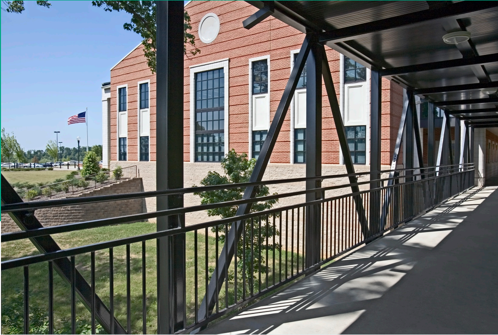
Steel-framed pedestrian bridges link the classroom wings on one side of the stream (visible here) with the assembly buildings on the other. The edge of the main entrance pavilion is just visible to the left of the classroom building.
