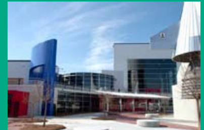
A plaza featuring the full size Saturn V model leads to ticketing and orientation with primary circulation at the second level. Painted insulated steel exterior panels here introduce NASA colors.
