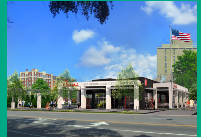
Arcades with floating canopies will create a strong presence for the modest building at a key corner. Cohen Carnaggio Reynolds specified more substantial materials: charcoal and white brick.
