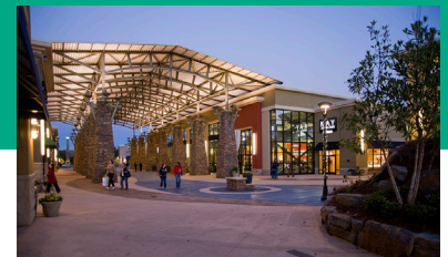
An area covered by a large canopy is used for concerts and other special events. Glass walls enclose the adjacent food court.
