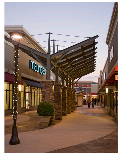
Circulation routes are designed like streets with native sandstone and steel canopies providing scale and some cover.
