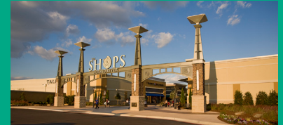
A compelling masonry and steel entrance gate fronting the open-air mall features monumental light towers.
