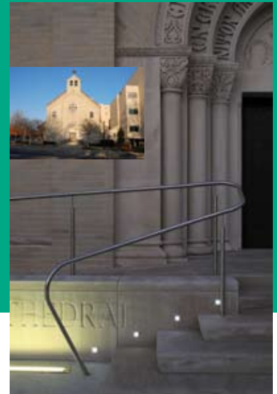
The church front before and a close view of the redone entrance shows how the steps were brought forward to make way for an access ramp behind.
