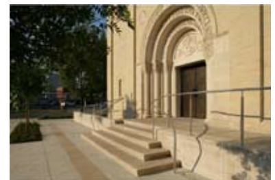
This view across the plaza shows the new main steps, the low wall that creates a new base for the building and the ramp leading off to the left.
