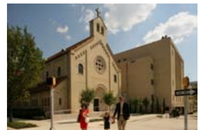
The outer plaza has a broad asymmetrical set of steps that resolve the grade change to the sloping city sidewalk.
