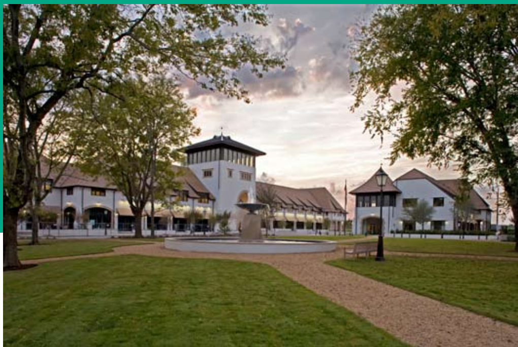
Hampstead's town center has begun to take shape with two mixed-use buildings facing the green square with its focal fountain. General contractor was Brasfield & Gorrie.
