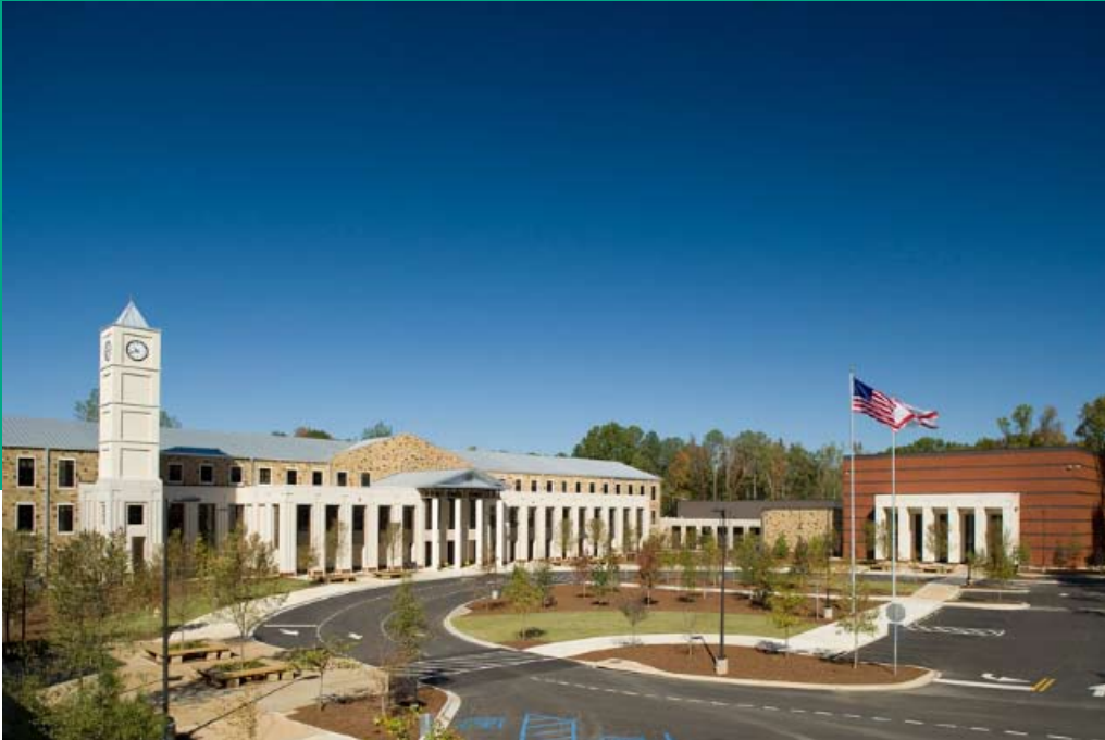
Hewitt-Trussville High School wraps around a new civic space punctuated by a clock tower. Ground-face masonry clads lower walls of the main wing with native sandstone above and red brick to distinguish the auditorium.
