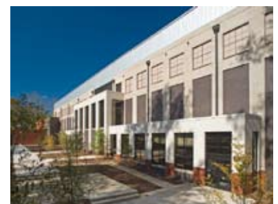
The bulk of the athletics wing that wraps one side of the front court is tamed by the classical colonnade pattern executed in two shades of ground-face blocks and a darker jumbo brick.
