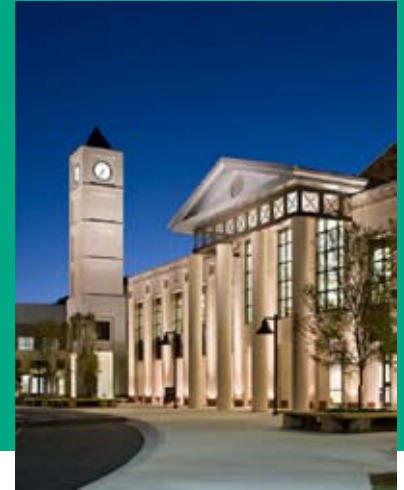
"I've always wanted to make a Doric portico of the most basic elements," says Neil Davis. The non-tapering poured concrete columns carry a Roman cross-patterned steel entablature.
