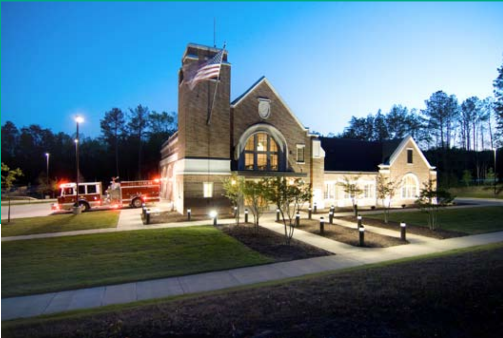
In this dusk view of Hoover Fire Station #2, the glow from the second floor commons can be seen through the large arched window with the wing to the right housing support spaces.
