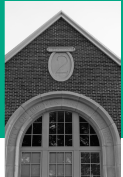
This black-and-white photo emphasizes the cast-stone detailing. The arch lettering reads "City of Hoover Fire Department."
