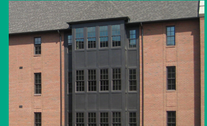
Brick, fiber-cement paneling and other exterior materials were selected for long-term maintenance benefits. Detailing helps give the buildings a domestic character.
