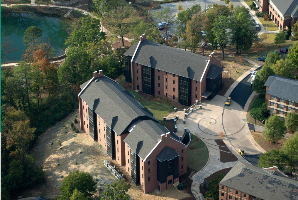
This aerial view shows the new Lakeview Residence Halls extending in an east-west orientation between existing dorms (right) and a new lake below. Behind projecting bays are the living rooms of four-bedroom suites.
