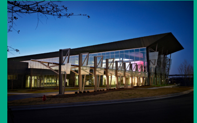
The transparency of the building along its U.S. 31 frontage is visible at dusk.
