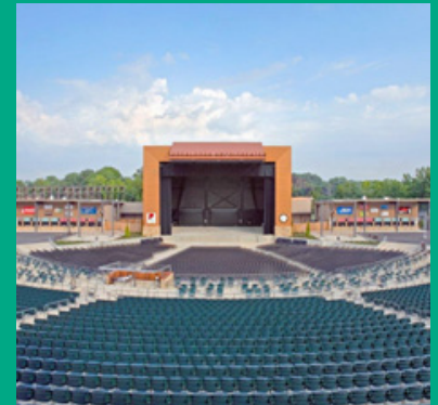
This daytime view shows the proscenium stage structure clad in painted metal panels flanked by support buildings. Exposed steel supports the porch-like structures that front these lower buildings. Photo by Lewis Kennedy
