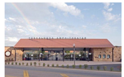
Expansive native sandstone walls, exposed steel framing and a metal panel roof topped by metal lettering welcome patrons. Photo by Lewis Kennedy
